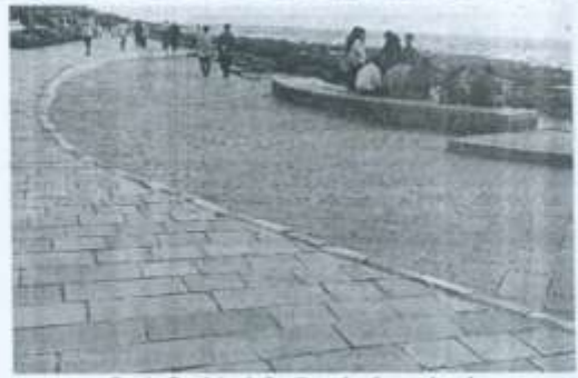
Bandra Bandstand after the redevelopment work
